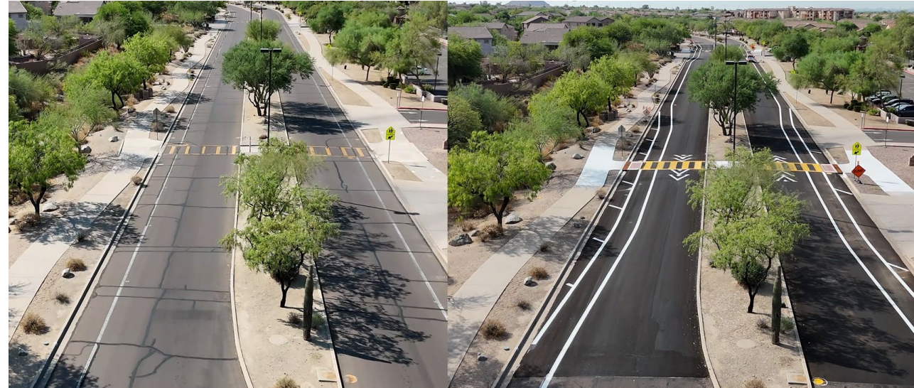
Las Sendas Elementary Raised Crosswalks
