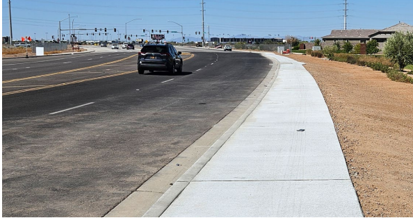
Williams Field Rd Sidewalk Installation
